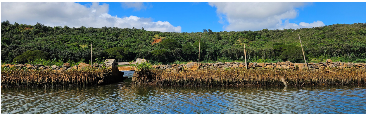
The kuapā with mākāhā and live mangrove wall that will be removed during the final stages of its restoration
