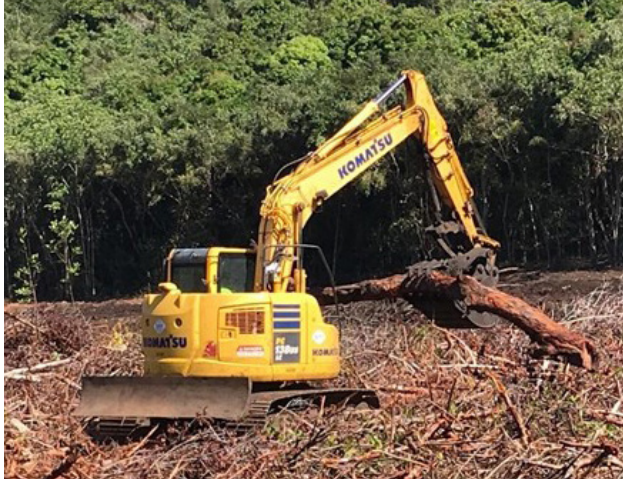
Figure 2-8. The use of heavy equipment was essential for mangrove removal in most areas in and around the pond (except for the kuapā).
